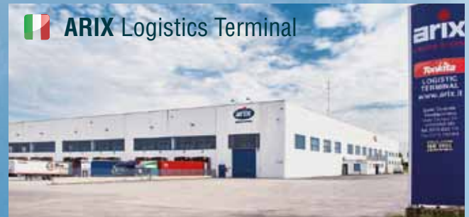
ARIX Logistics Terminal Piattaforma Distributiva - Logistics Terminal Total Area: 48.000 mq - Buildings: 10.000 mq
