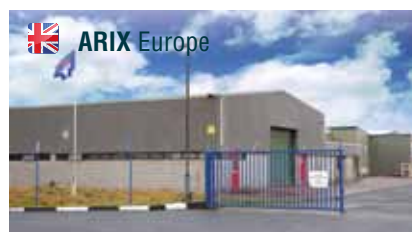
ARIX Europe Unità Logistico-Commerciale UK, Irlanda e Nord Europa Northern Europe Sales and UK & Eire Distribution Total Area: 48.500 mq - Buildings: 3.000 mq
